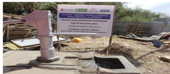
Abandoned water well in Ex-airport after rehabilitation
