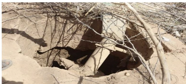
Abandoned water well in Ex-airport before rehabilitation
